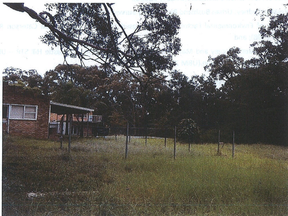
Plate 5: Existing house and garden with native bushland to east (RHS photo)
